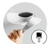
trimless installation in plasterboard
